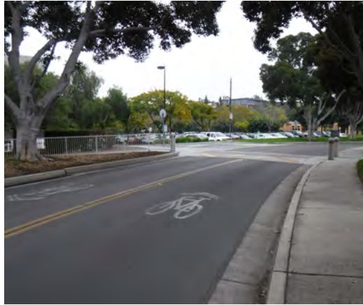
A bike route with shared lane marking (sharrow), UC Irvine campus.
