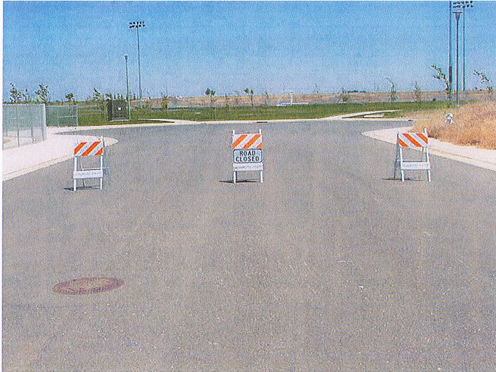
Configuration of barricades and R11-2 sign ("Road Closed") at the closure.
