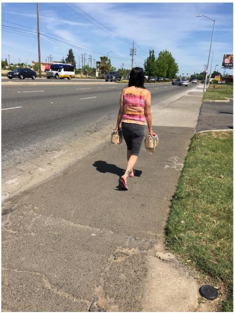
There are no bike lanes along this segment and existing sidewalk is attached and mostly with rolled curbs and is not ADA compliant.
